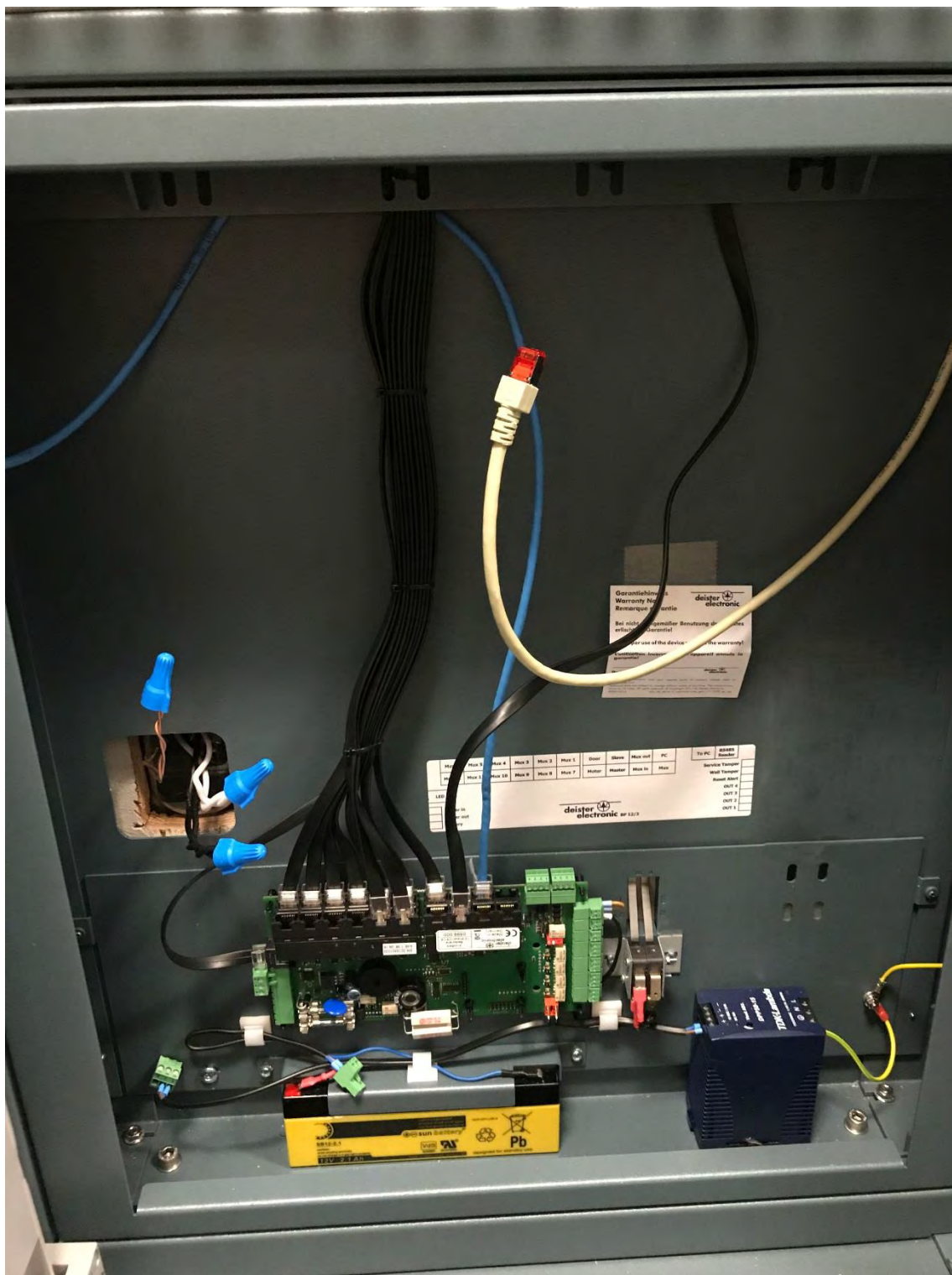
PICTURE OF HARD-WIRED POWER (KT-12 Module Cabinet)
