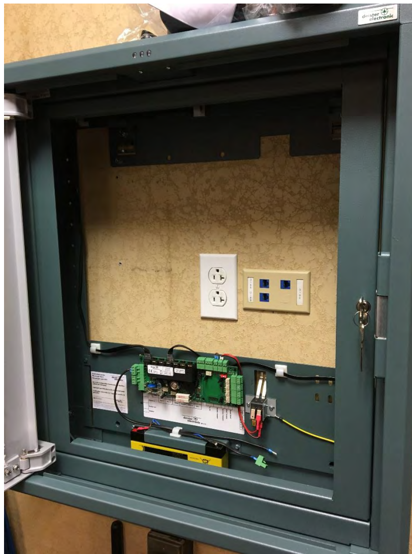
PICTURE OF POWER OUTLET FLUSH MOUNTED FOR 4-MODULE CABINET
